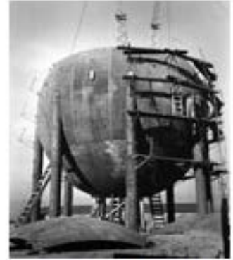
Courtesy of Chuck Dasey The "Eight Ball" under construction
